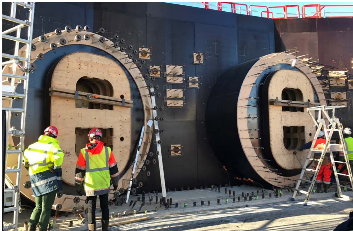
The entry points of the ITER Neutral Beam Injectors at the second floor of the Bioshield, Tokamak Complex, December 2016, © Engage
