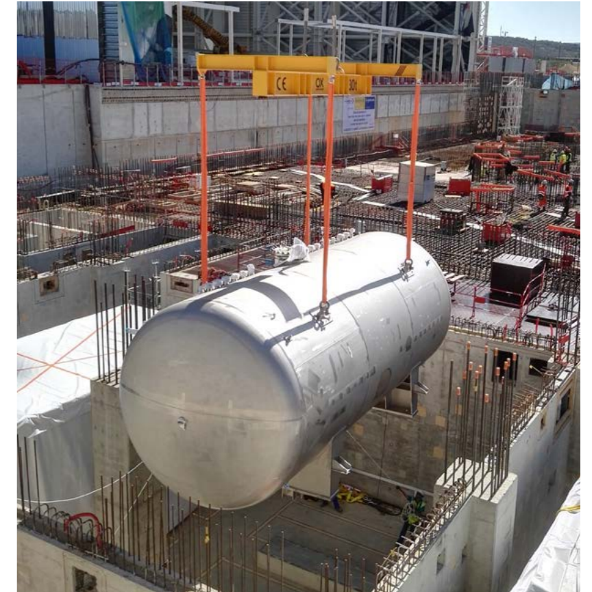
Transferring one of the bigger water detritiation tanks weighing approximately 20 T in ITER's Tritium building
