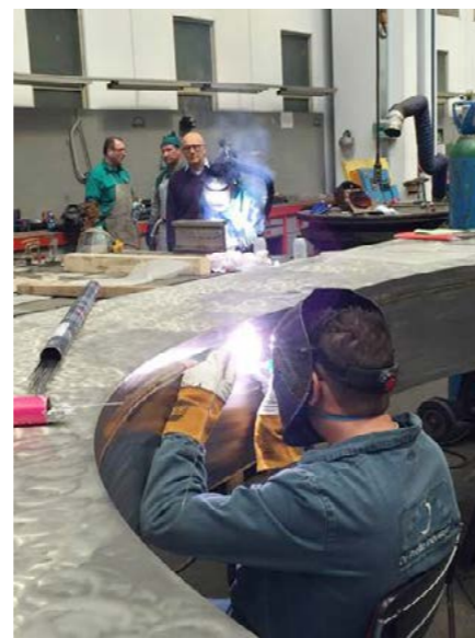
Welding of the MITICA Vacuum Vessel in progress
