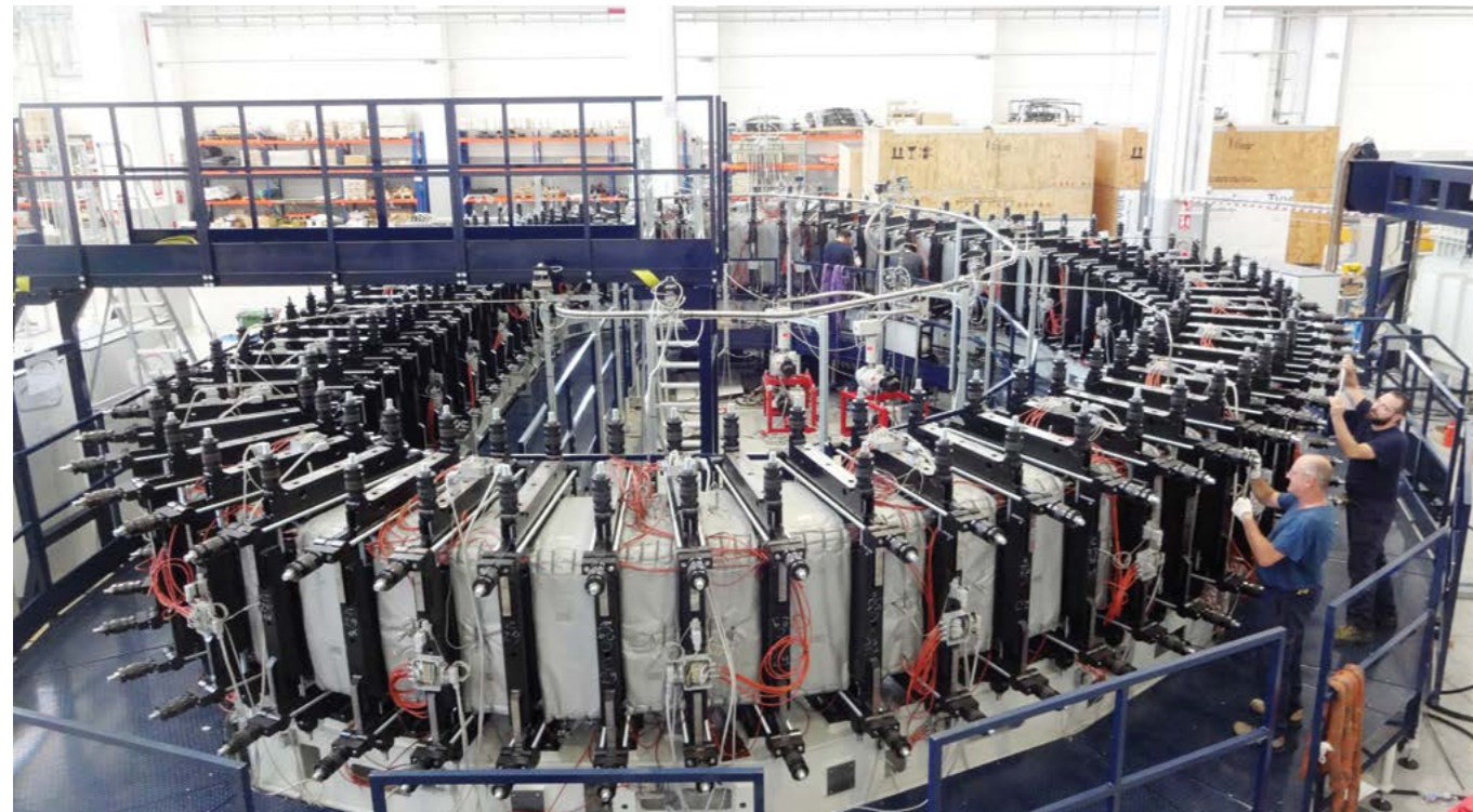
Compacting the inner-core of the first Toroidal Field coil, ASG Facility, La Spezia, Italy
