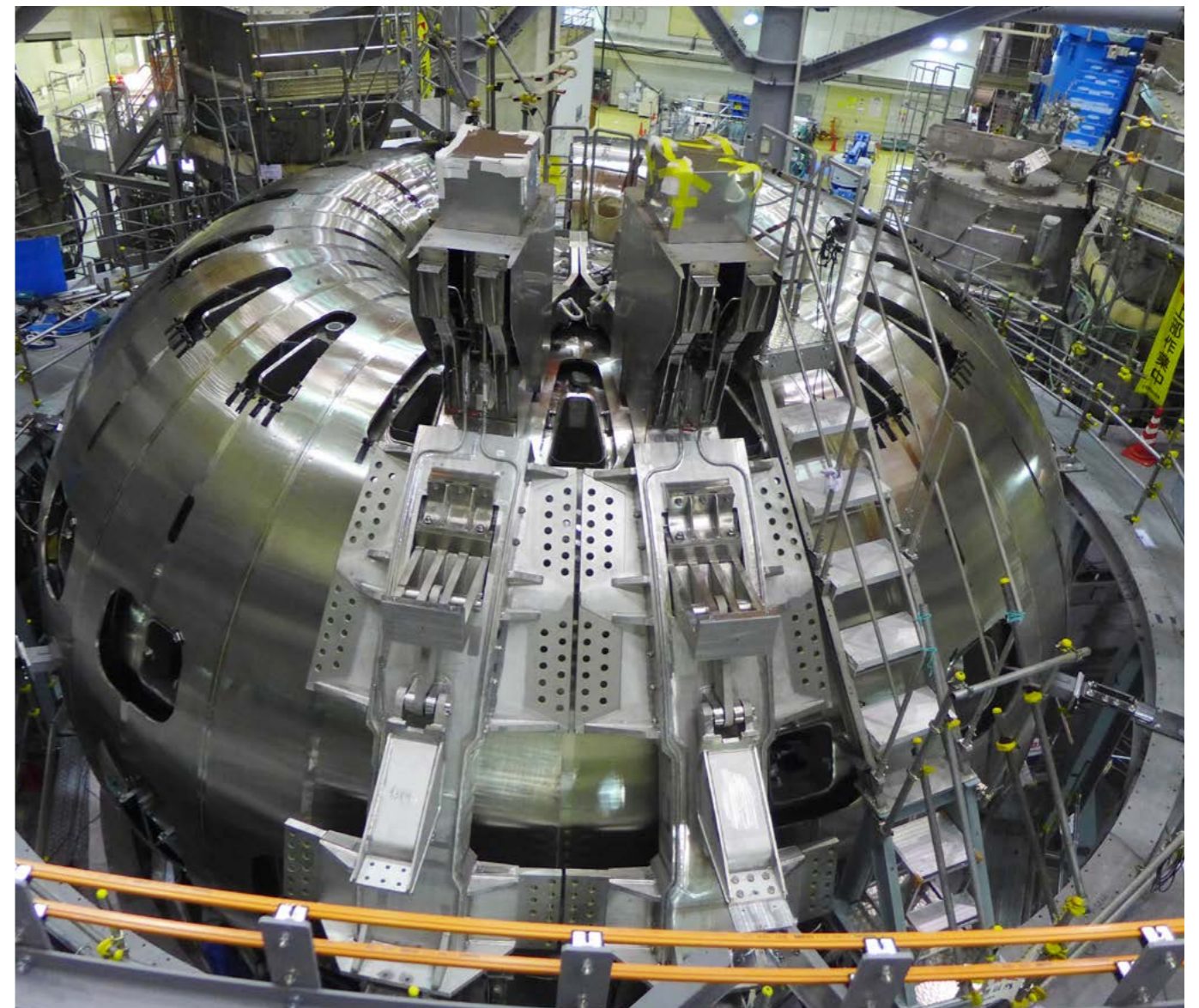
The assembly has started: the first two of JT-60SA's TF coils are in place in the Tokamak
