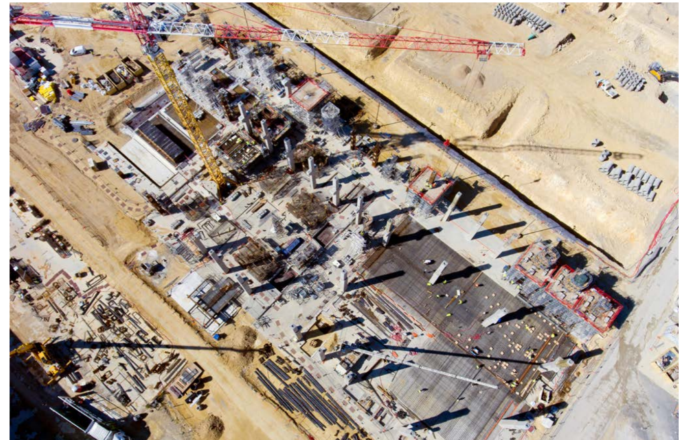
ITER Worksite - Cryoplant Building - October 2016
