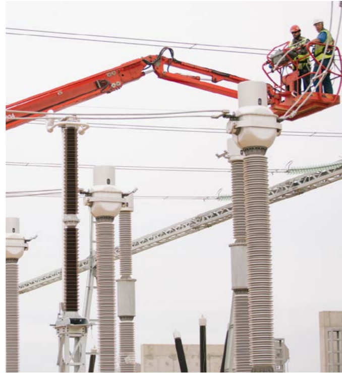
Technical teams checking the cabling where the ITER substation will be connected to France's grid to receive 400 kV, November 2016, © LNM
