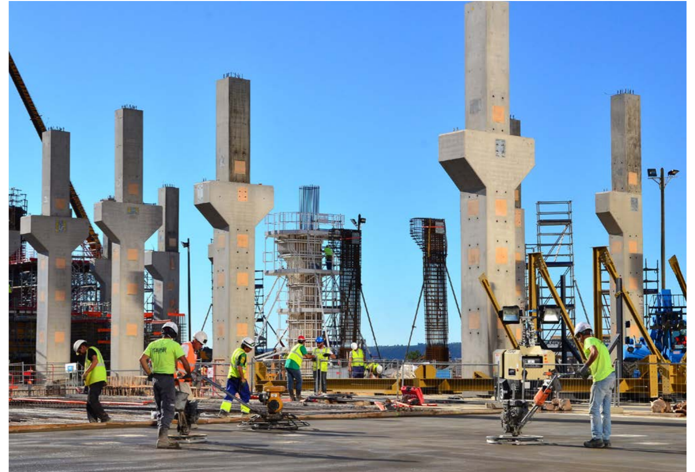
Construction works in progress at the ITER Cryoplant, November 2016, © ITER IO
