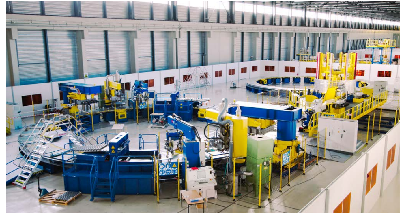
Winding tooling at the Poloidal Field coils Facility where cleaning, sandblasting, bending, insulation and wrapping of the conductor will be performed, Cadarache. August 2016
