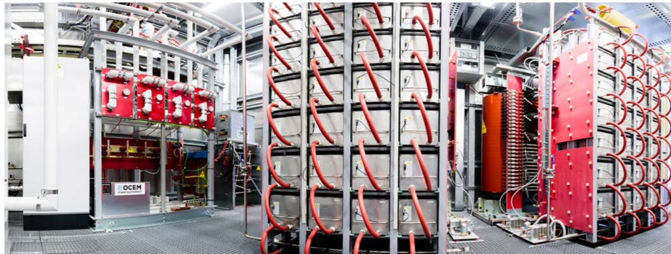
ISEPS of SPIDER equipment fully installed and tested inside the High-Voltage Deck
