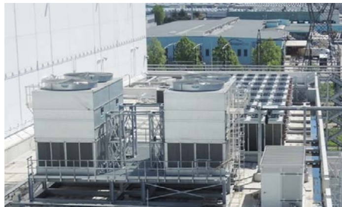
Cooling towers and heat exchangers on the roof of the Neutral Beam Test Facility, Padua, Italy
