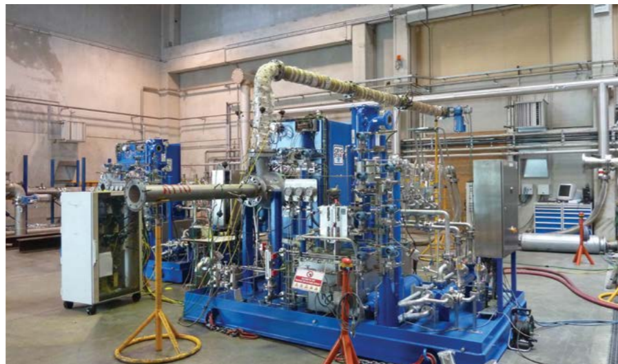
Turbo booster turbine able to generate 500 KW of cooling power fully assembled for testing at Cryostar
