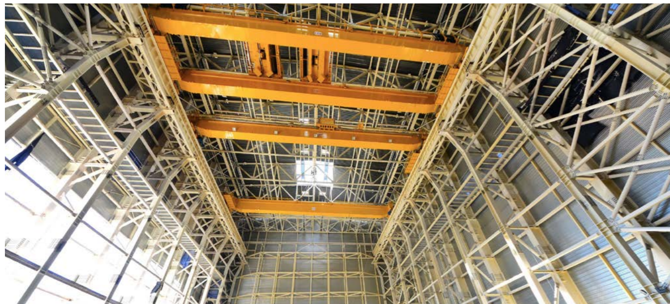
The second girder of the cranes operating in the Assembly Hall has arrived at the ITER site, March 2016 The four girders of the cranes that will lift the bulky ITER components have been installed in the Assembly Hall, July 2016, Cadarache © Engage The impressive monster crawler crane that was used to help with the lifting operation, July 2016, Cadarache The two auxiliary 50 T cranes at the Assembly Hall, November 2016, © Engage
