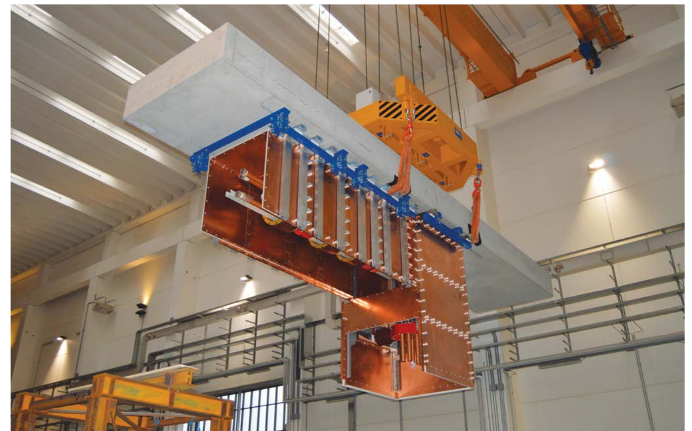
Part of the 35 m long transmission line which is connected to the SPIDER vessel
