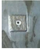
Figure 6 metal plate with threaded hole welded to a component to install a survey target nest
