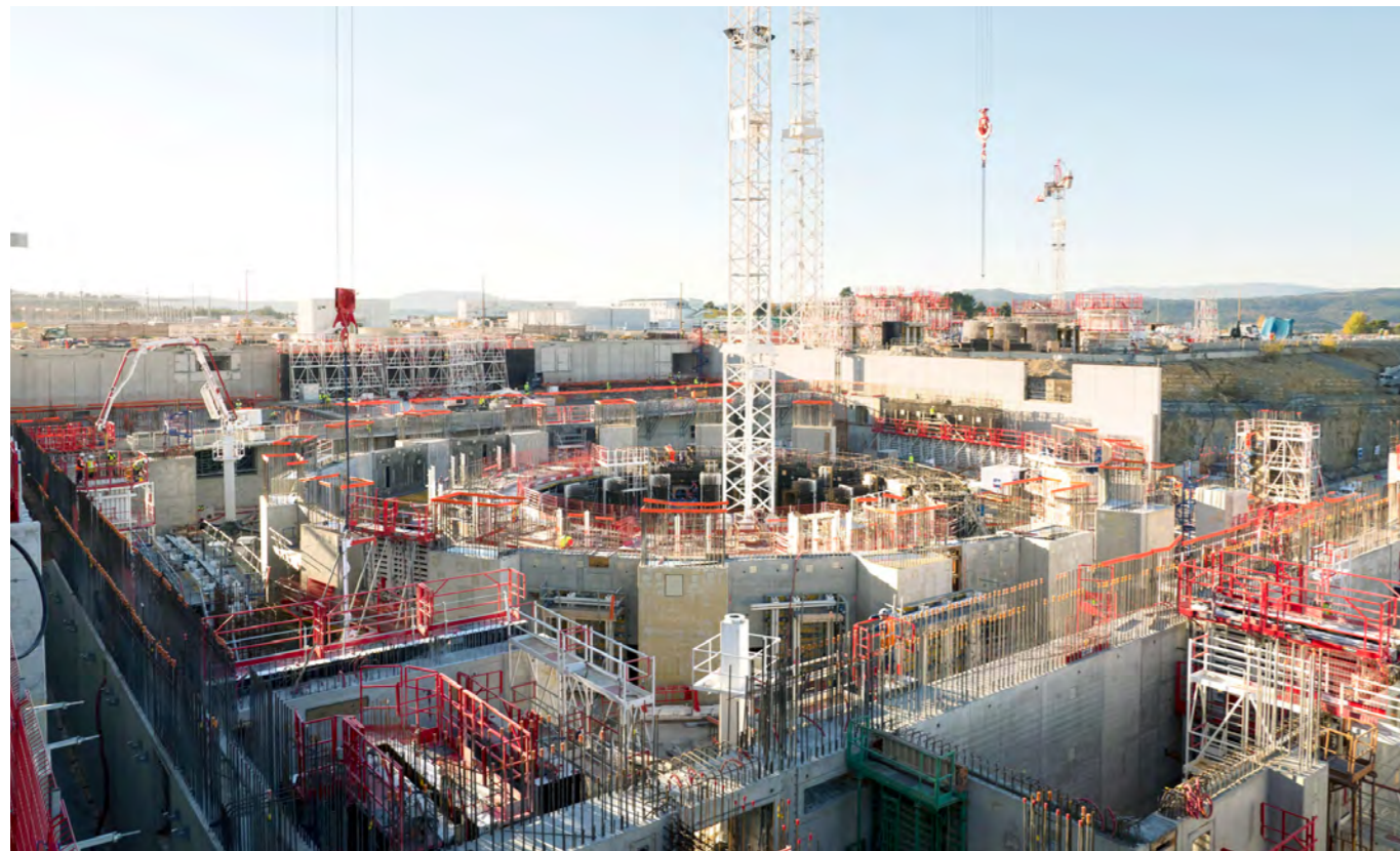
The Tokamak Building seen from the south of the Tritium Building – November 2015
