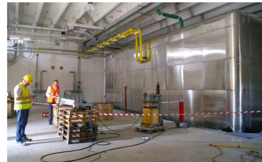
During the acceptance tests of the SPIDER High-Voltage Deck (HVD) at the Neutral Beam Test Facility (NBTF) at the Consorzio RFX site in Padua, Italy
