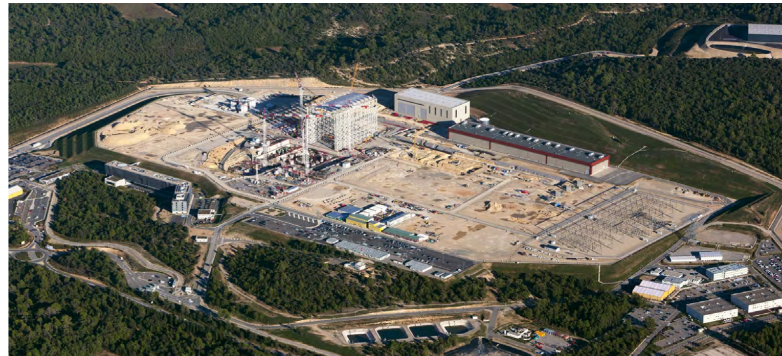
Aerial view of ITER construction site, September 2015, ©MatthieuColin.com
