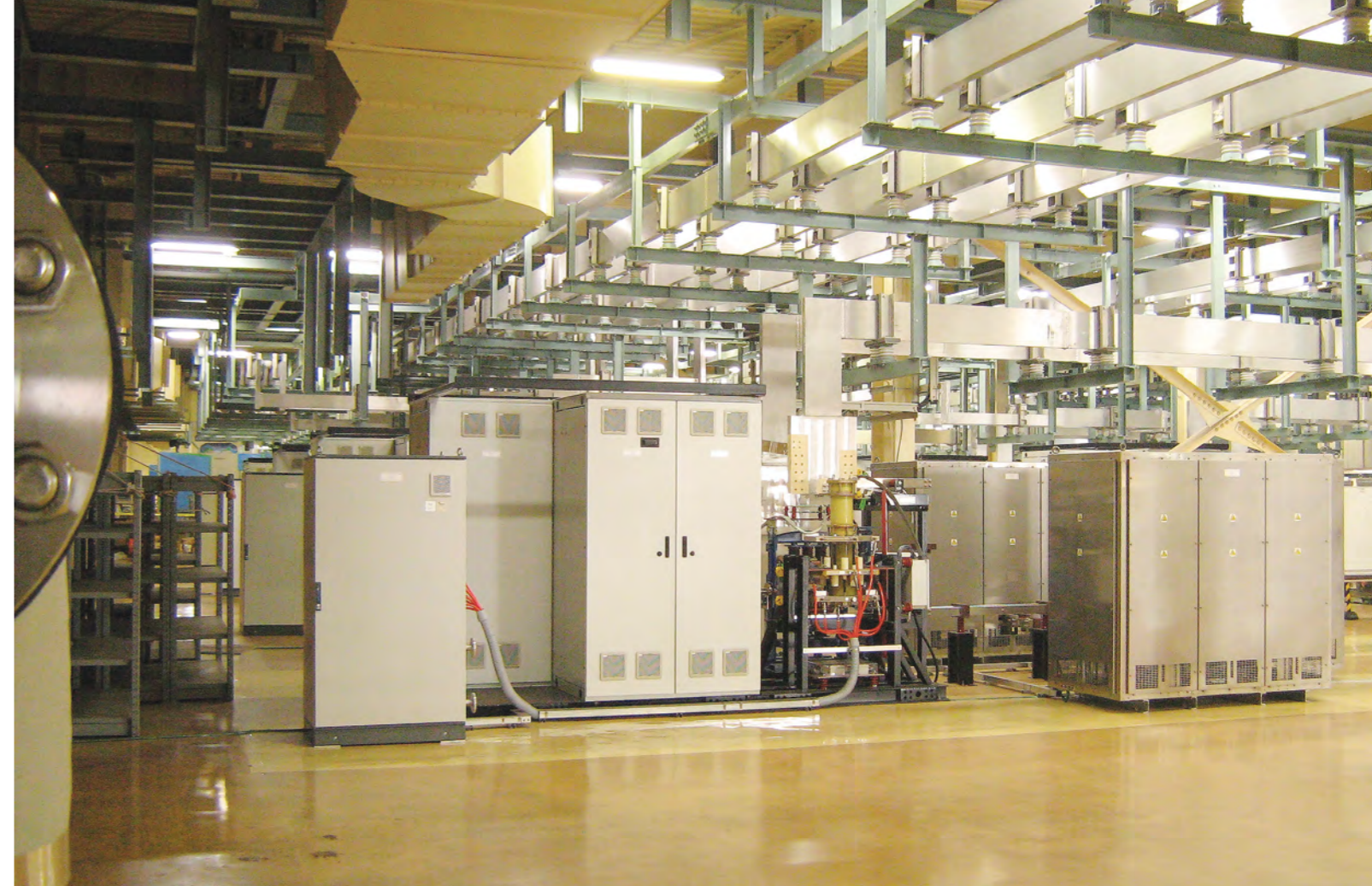
One of the 13 QPC units after installation in Naka, Japan
