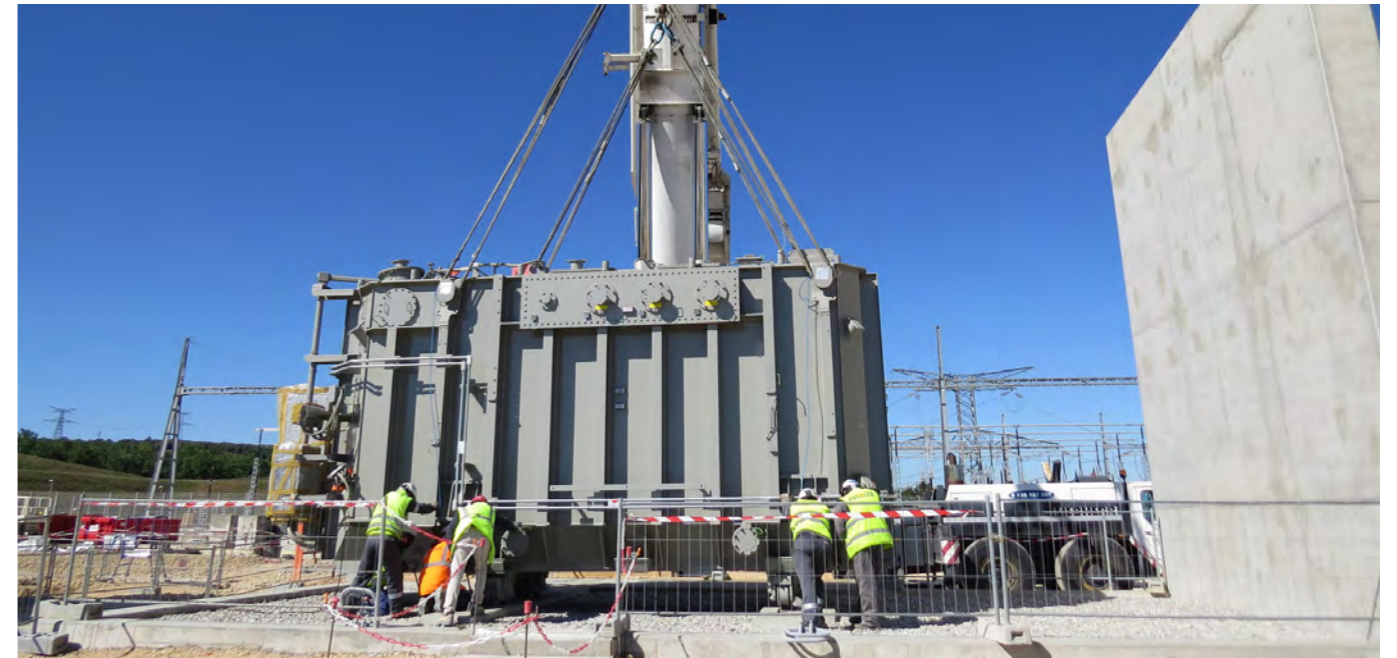
The two transformers being installed on the ITER site
