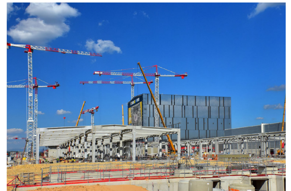
Installing the steel structure of the Magnet Power Conversion Buildings, ITER construction site, July 2017 © ITER IO
