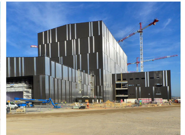
01 – Installing the first pieces of equipment inside the ITER Assembly Hall, September 2017 © LNM-Engage
