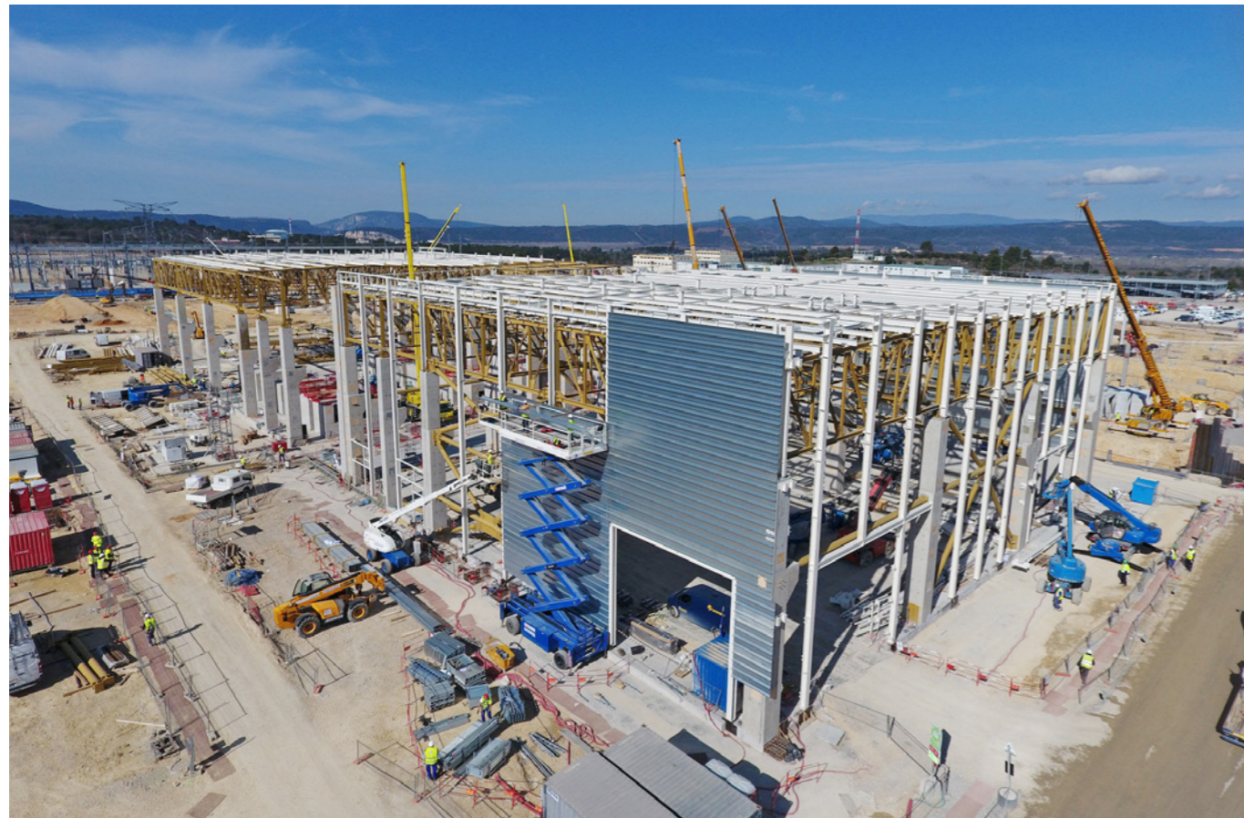
Cladding operations starting early in the year at the ITER Cryoplat, April 2017 © LNM
