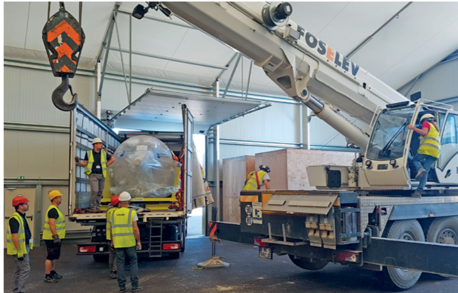
Delivery of cryopump to ITER site, Cadarache © F4E
