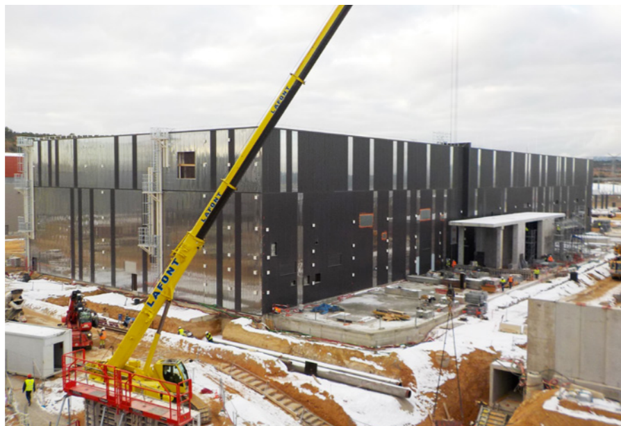
Final works at the ITER Cryoplat before the first tanks get installed, December 2017 ©Engage
