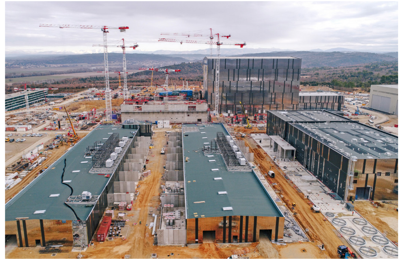
(L-R) Aerial view of the two ITER Magnet Power Conversion buildings and the ITER Cryoplat, December 2017 © SNC Engage
