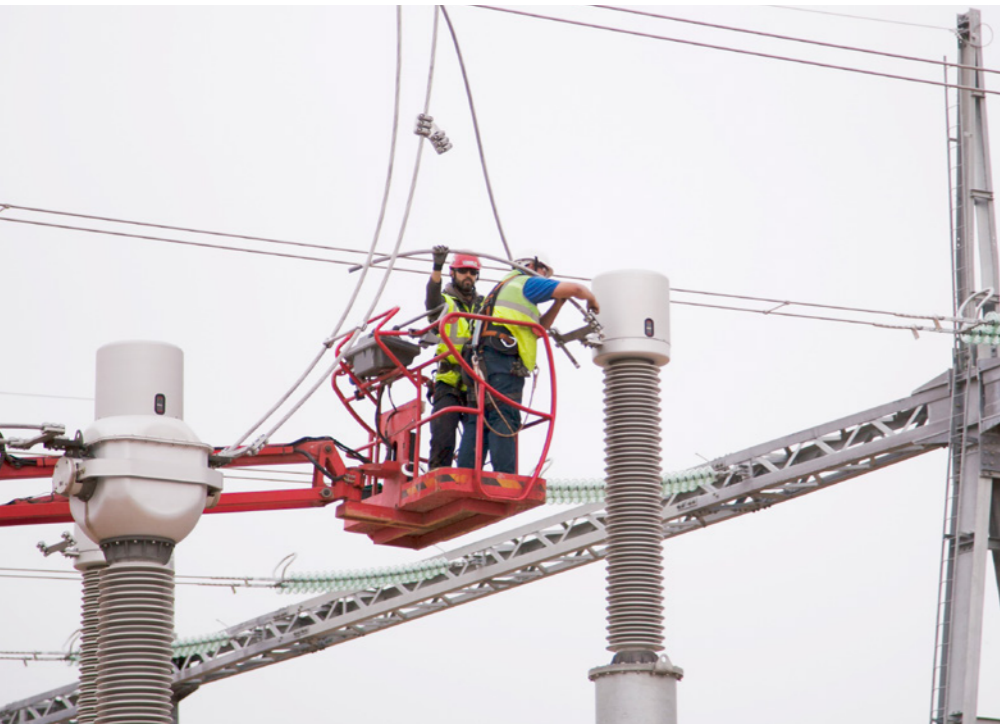
Technical teams on-site cross-checking cabling before the ITER site is connected to the grid © SNC Engage
