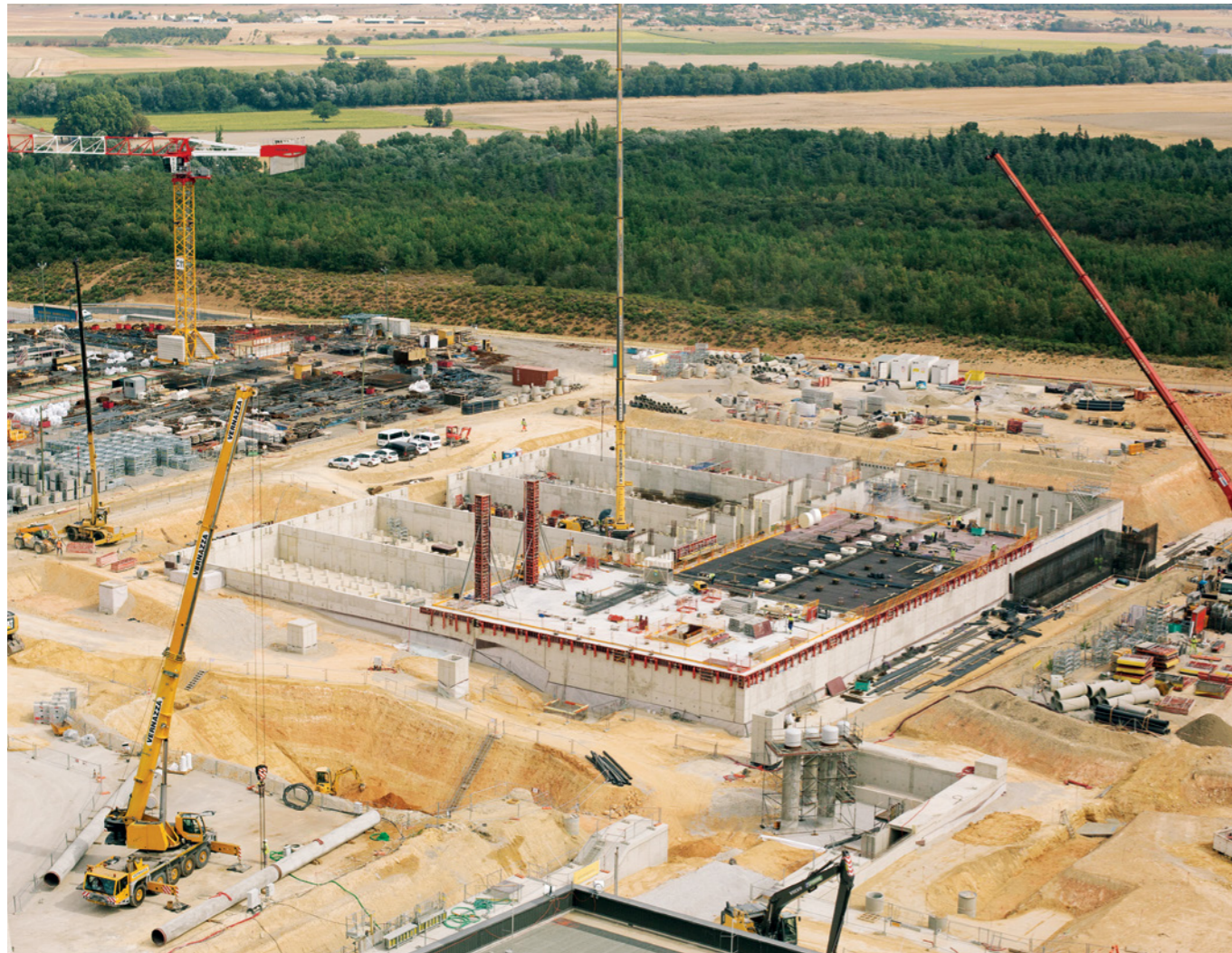
Aerial view of the works in progress at the area of the water basin and cooling towers, ITER construction site, September 2017 © LNM-Engage
