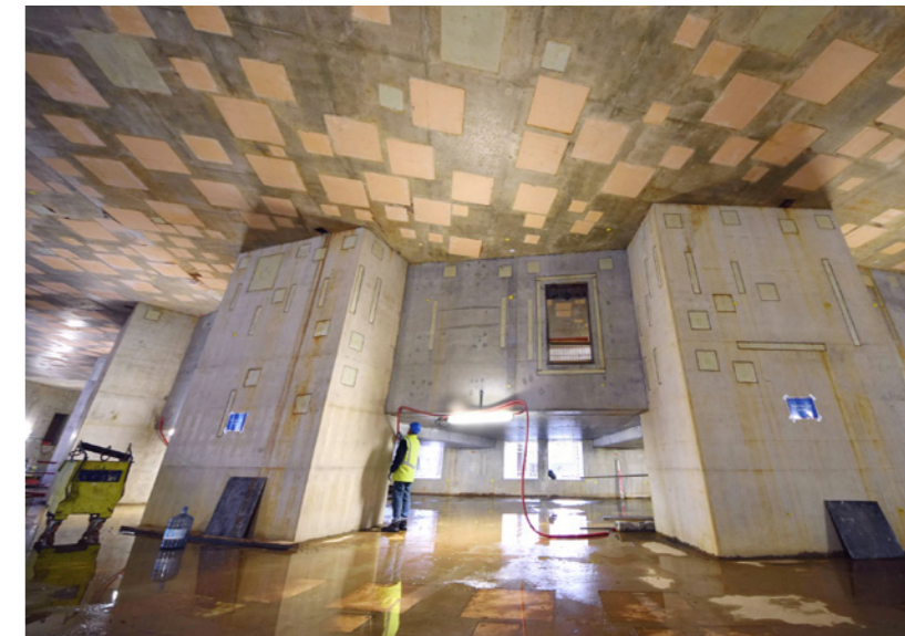
Various embedded plates installed on the level above, Tokamak building © ITER IO
