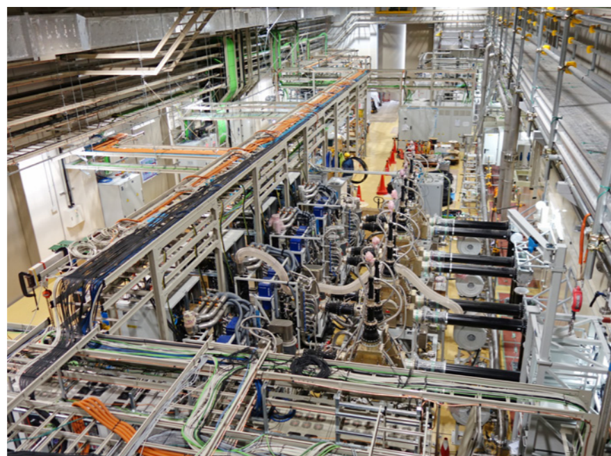
Top view of the Radiofrequency Area of the LIPAc facility, Rokkasho, Japan
