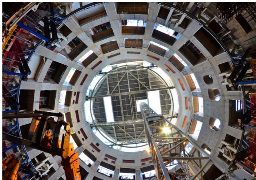
View of the ITER Bioshield lid positioned 30 m high ©ITER IO
