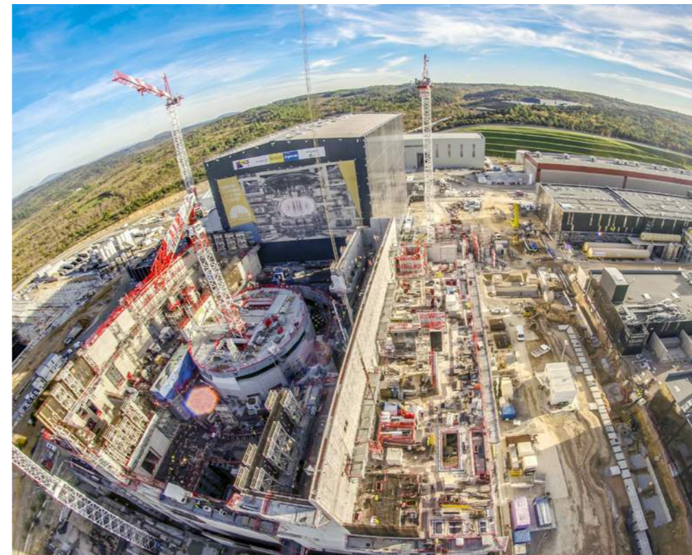
Aerial view of the Tokamak Complex © ITER IO
