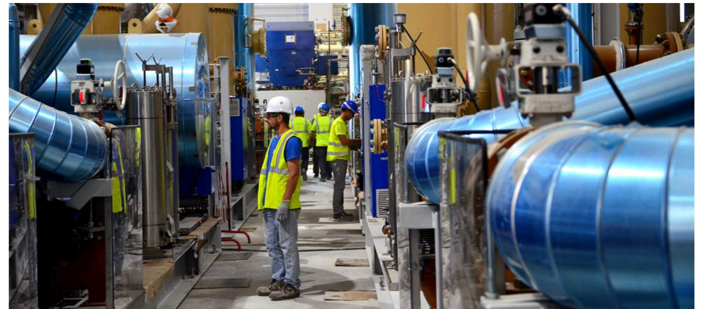
Technicians checking the installation of compressors in the ITER Cryoplant
