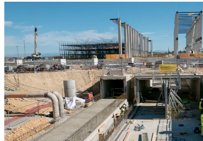
Works advancing in galleries © SNC Engage
