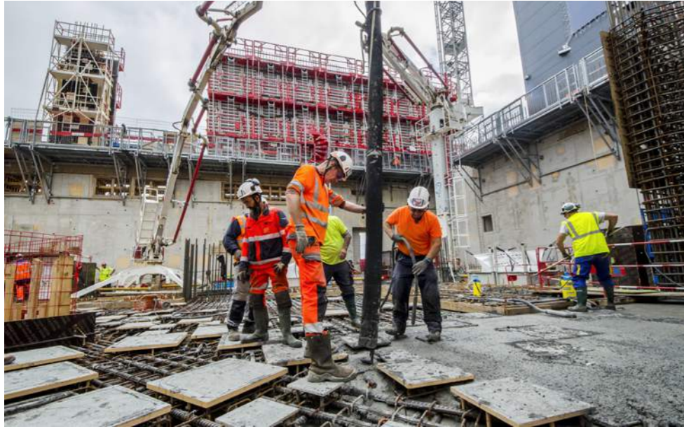
Pouring of borated heavy concrete in the area of the cooling water exchangers in the Tokamak building © ITER IO
