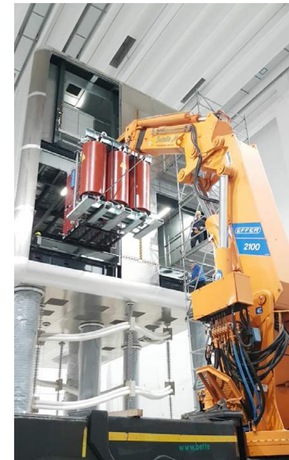
Installing in MITICA's High Voltage Deck, produced by Siemens, the ion source power supply equipment manufactured by OCEM PE.
