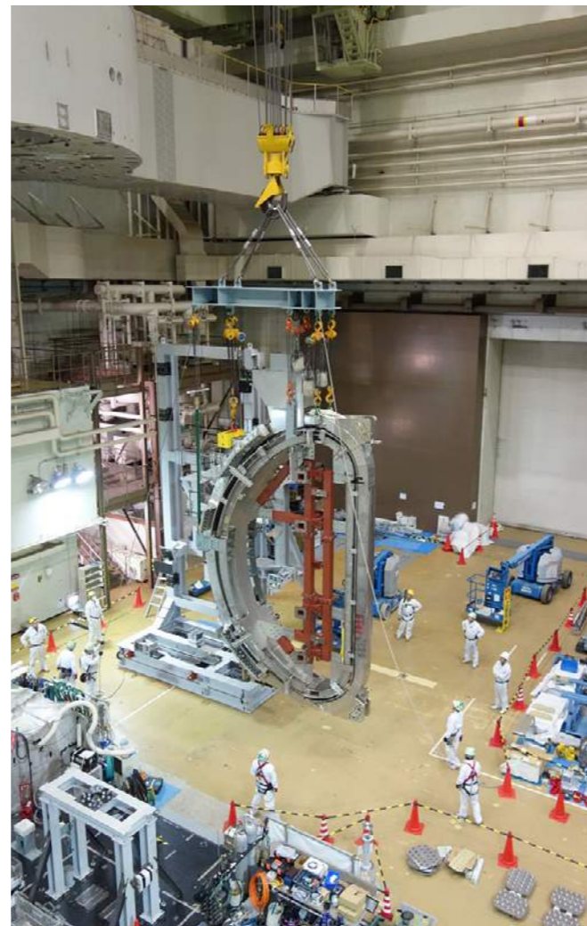
The pre-assembled sector comprising TF coil, final vacuum vessel sector and its thermal shield being lifted for installation © QST
