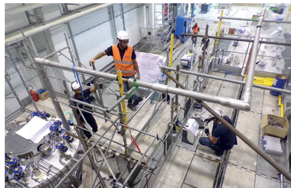
Connecting the main cold box, on the left, with the auxiliary cold box, on the far right, with the help of cryolines, ITER Neutral Beam Test Facility, MITICA, Padua, Italy
