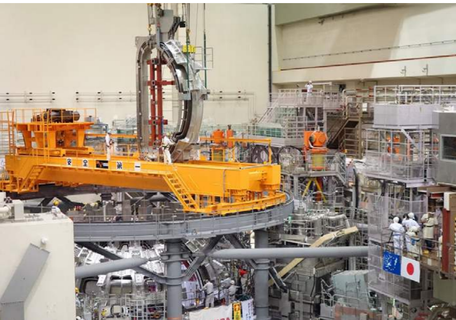
The last TF coil being installed in JT-60SA (Photo courtesy of QST).
