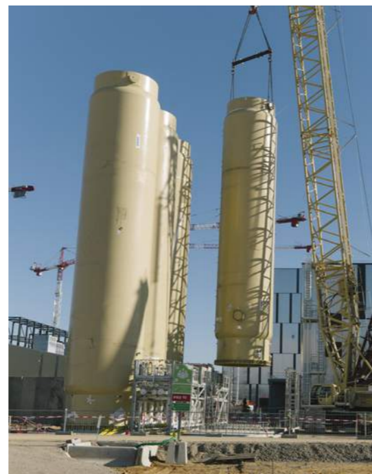
Finalising the installation of Europe's cryogenic tanks on-site, ITER Cryoplant © SNC Engage
