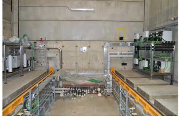
General overview of on-going installation of the vacuum system inside the SPIDER bio-shielding
