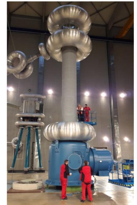
The installation of the High Voltage Deck inside the MITICA High Voltage hall, October 2017. © Consorzio RFX
