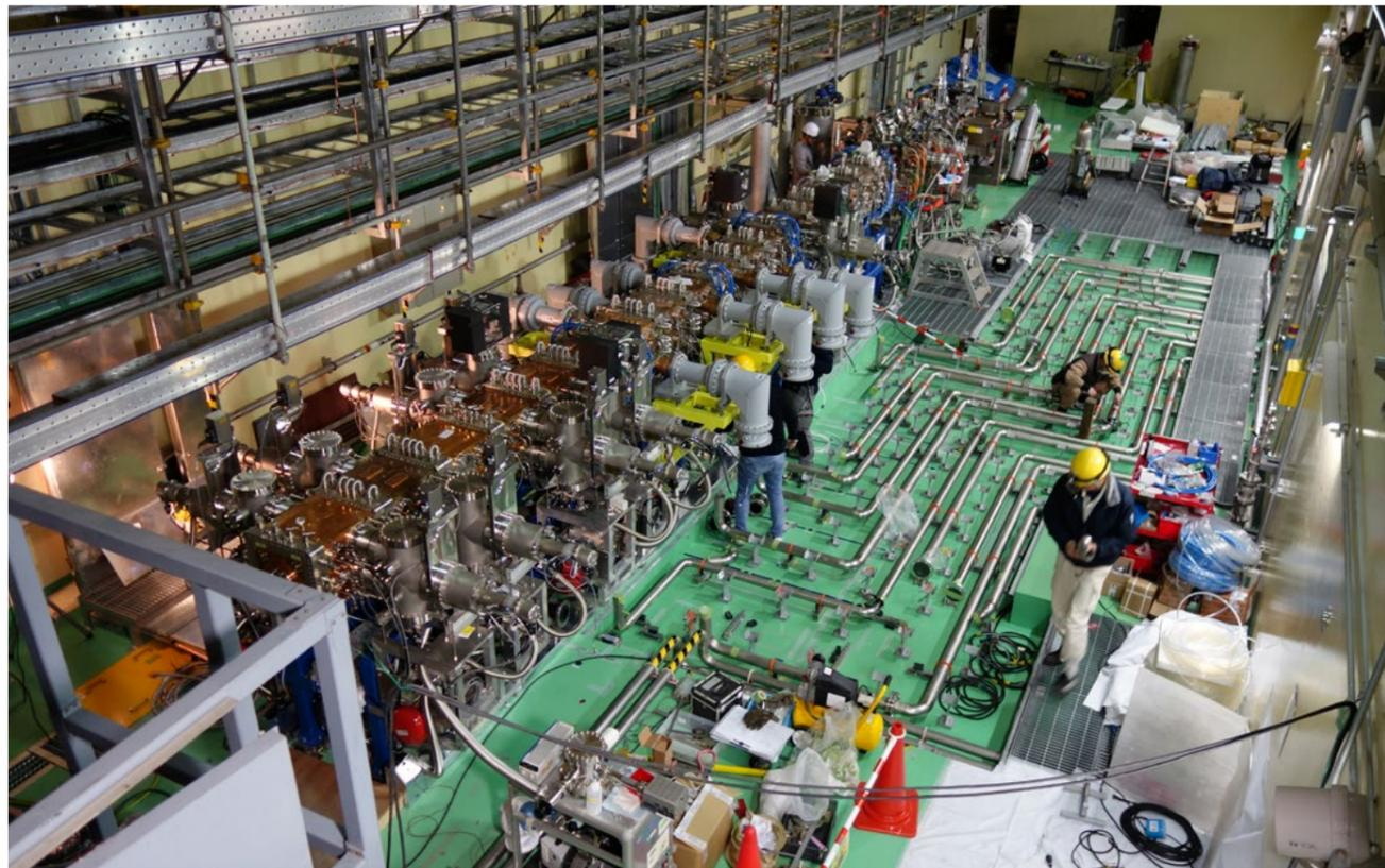
Top view into the LIPac accelerator vault during the installation of the cooling loops for the "Radiofrequency Quadrupole", Rokkasho, Japan
