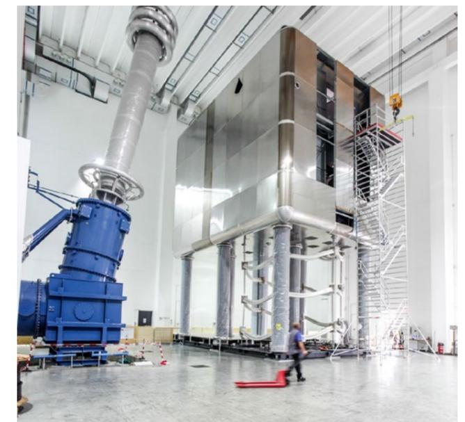
The installation of the High Voltage Deck inside the MITICA High Voltage hall, October 2017. © Consorzio RFX
