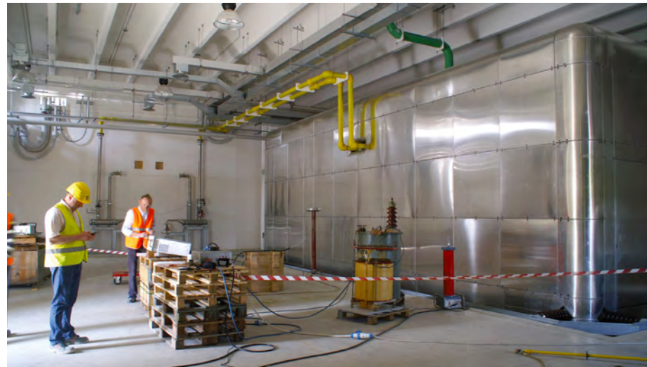
During the acceptance tests of the SPIDER High-Voltage Deck (HVD) at the Neutral Beam Test Facility (NBTF) at the Consorzio RFX site in Padua, Italy.
