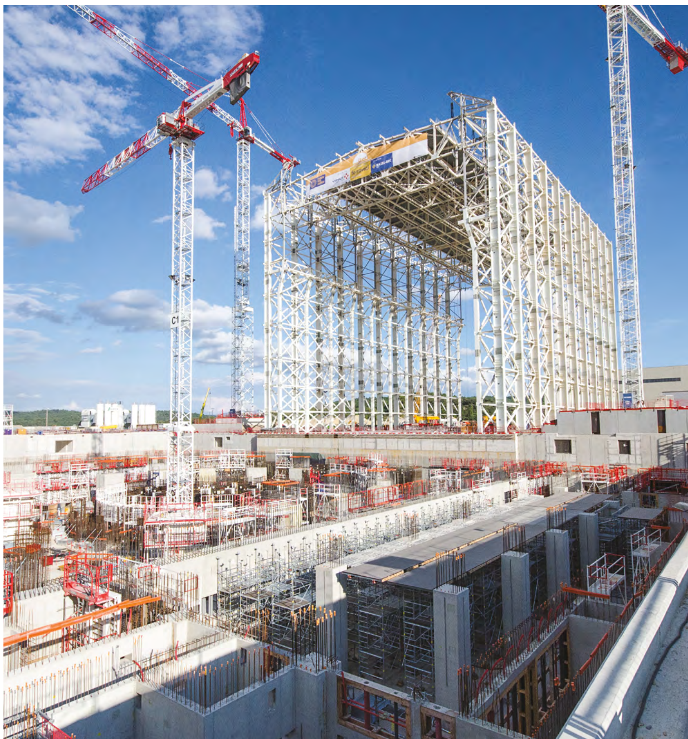
The ITER Assembly Hall building
