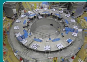
Completion of assembly of cryostat base in the Torus Hall at the Naka Fusion Institute
