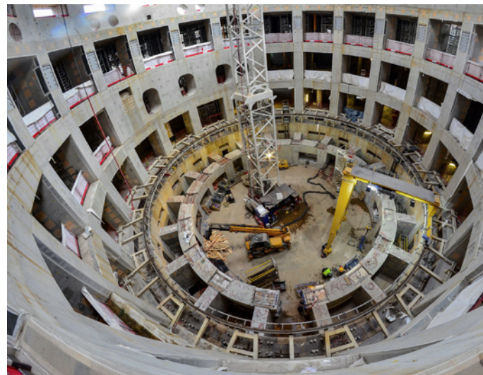
The ITER crown, a solid base ring and its 18 radial walls able to support the load of 23 000 t, has been completed. The works have been financed by F4E, responsible for the construction of the infrastructure and facilities on-site.
