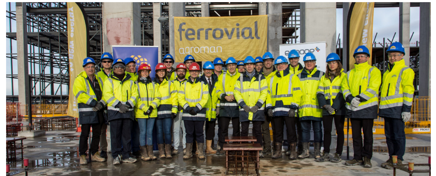
The handover of the cooling tower zone from F4E to the ITER Organization, ITER Construction site, December 2018, Cadarache, France. Now the ITER team will supervise the installation of equipment sent by India © ITER Organization
