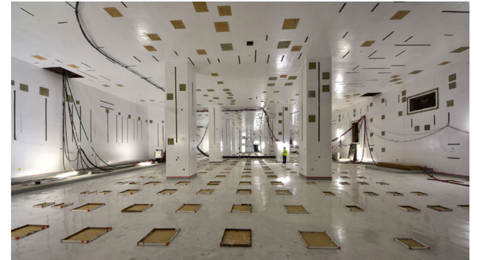
The first level of the Diagnostics building ready for handover to contractors for the beginning of systems installation. The embedded plates visible on all surfaces will allow contractors to attach the supports required to install various systems. © ITER Organization
