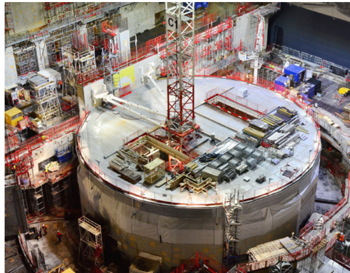
The lid covering the fully-completed bioshield, Tokamak building, ITER construction site, Cadarache, France. The works have been financed by F4E, responsible for the construction of the infrastructure and facilities on-site.
