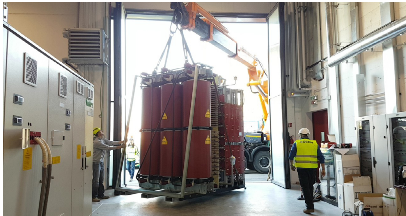
The power supply for the Residual Ion Dump (RID), manufactured by OCEM PE, financed by F4E, has been delivered to MITICA - the second experiment of the ITER Neutral Beam Test Facility, Consorzio RFX, Padua, Italy. On the left, the Acceleration Grid Power Supplies Conversion System, produced by NIDEC ASI, financed by F4E.
