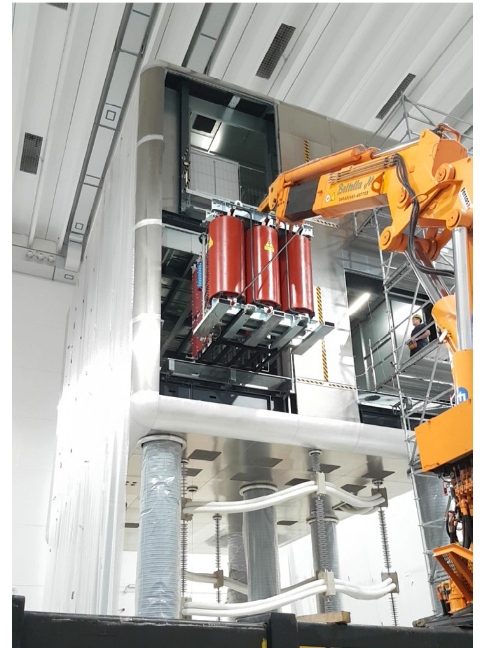
Installing in MITICA's High Voltage Deck, produced by Siemens, the Ion Source Power Supply equipment manufactured by OCEM PE.
